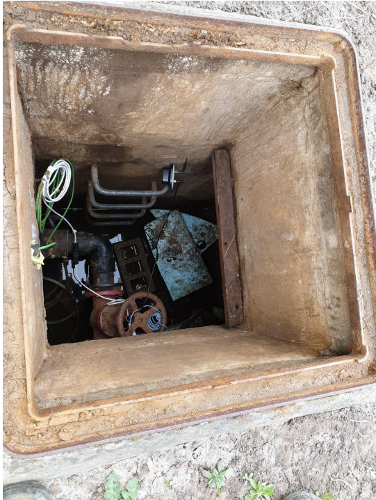
Exterior Manhole under metal plates
